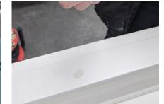
Apply several coats of matched colour Teknos Aquatop 2600 paint over the sanded area of filler. Touch up paint can be partially diluted with a small amount of clean water to achieve a smoother finish. More coats of a diluted paint will be required to cover the damaged area, however this will ensure a much smoother finish.
