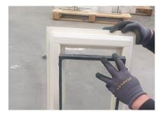
Place 2 glazing spacers into the glazing cavity at the bottom, with the centre of each spacer approximately 100mm in from the corners. Then, lift the replacement glass unit into the window aperture and place it onto the glazing spacers, ensuring equal spacing all around the glass. Additional glazing spacers may be fitted to ensure the glass remains central.
