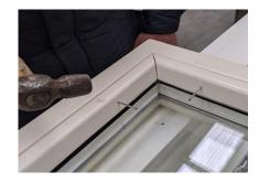
Once the silicone has been applied, the silicone area should be sprayed with a water and soap solution to allow the silicone to be worked. We recommend a strong mix approximately 10–20 parts washing up liquid to 80–90 parts water will provide the best finish.
