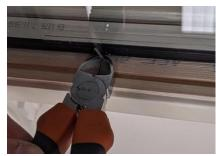
The glass should now be removed from the inside, lifting the entire unit out of the frame. Remove any remaining silicone from the glazing up-stand and glazing bead to leave a clean surface.
