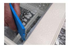
Silicone sealant should now be liberally re-applied between each bead and the glass using a Silicone Gun around the full perimeter of the unit. Silicone should be applied both inside and out to ensure a weatherseal.
