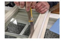
A chisel can then be carefully inserted and used to prise the bead off completely. Take care not to flex the bead too much or cracking may occur. Repeat this process for the remainder of the beads.
