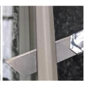
Remove all timber glazing beads, starting with the longest.
