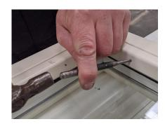
Once the area is sprayed but before the silicone has set, a silicone finishing tool can be used to scrape away excess silicone and force the silicone into the groove between the bead and glass.
