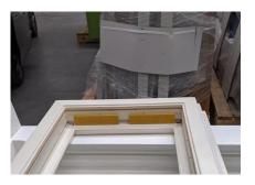
Once the glass unit is sat centrally within the aperture, the beads can be refitted. Any beads damaged or cracked during removal can be replaced with new beads at this stage. Beads should be refitted starting with the shortest one first, then proceeding to the longer ones. When a bead is placed into position ensure it is providing compression on the glazing to
