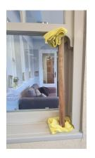
Locate the bottom of the balances, found inside the balance channels at either side of the window. A threaded hole should be visible at the bottom of each balance. Take the Spiral Balance Removal Tool and screw the threaded end of the tool into the bottom of the balance to be replaced.
