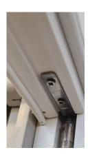
Before proceeding, ensure the support timber is taking the weight of the sash then undo the screws securing the balance foot to the sash and gently pull down on the spiral balance tool to extend the spring inside the balance out of the bottom by about 150mm.
