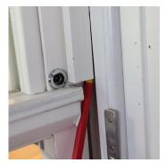
Now the top sash can be removed. Follow the instructions for the removal of the bottom sash in steps 2 – 4 including the use of a support timber. Note however that there will be no fixing screws holding the foot to the top sash.
