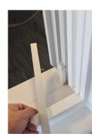
Slide the top sash down by 100mm to allow access to the top section of parting bead. This can be easily removed by inserting a flat head screwdriver between the bead and the frame and carefully levering the bead away from the frame. Place all the parting beads to one side for refitting once the sash has been replaced.
