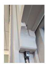
The upper sash can now be lifted out of the frame and into the property, removing the support timber.
