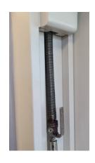
Once the balance spring is extended by around 150mm, tilt the foot back until it is touching the spring. This will prevent it from re-engaging as the spring slides back up the channel. The spring should now be gently allowed to retract back up and into the balance channel. Once the spring has been fully retracted inside the balance and is no longer connected to the sash the balance tool can be unscrewed from the bottom of the balance. Repeat the process for both sides of the sash.
