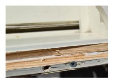
As Bereco Cill Extensions are glued into the cill groove for extra strength, there will be some timber from the cill extension left behind within this groove. Some timber may also be stuck to the window below the groove. All remaining timber from the cill extension should be carefully removed with a sharp chisel, taking care not to cut into the window itself.
