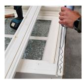
Using the Opti-Joint XP flexible sealant, apply a small bead along the top joint where the cill meets the window frame. Using a silicone finishing tool or similar item, scrape off any excess leaving a small bead of flexible sealant to seal the joint. Allow 15 mins for the opti-joint xp to partially set & apply 2 coats of paint.
