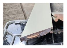
Working on one piece at a time, install the cill extension onto the window (See Installing Cill Extensions section of this guide for more information). Insert the biscuit to hold the joints flush, then install the next piece of cill extension. Metal fixing plates should be fixed across the join on the underside of the cill to prevent the joint from opening up during seasonal movement.
