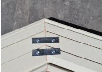
The cill joint should now be sealed with opti-joint xp flexible sealant, allowed to cure for 15 minutes, and then touched up with paint to finish (paint is supplied with the original order, more can be ordered on request).
