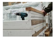
Screw the cill to the frame using the pre-drilled holes and 45mm screws, being careful not to over tighten screws causing the timber to split.
