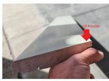
TIP: When measuring and marking the length of the bay cill ensure you mark and measure on the knuckle of the cill extension and not the back side of the cill tongue.
