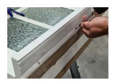
Using Opti-Joint XP flexible sealant, apply a bead both within the cill groove on the window and to the section of timber just below the cill groove as seen in the pictures below.
