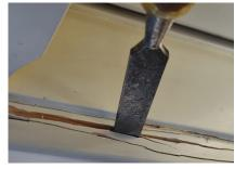
Once the majority of the cill extension is removed you will have access to the anchoring screws, these should now be removed.
