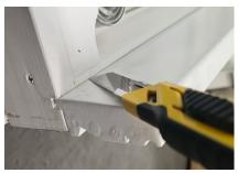
Using a sharp chisel cut across the cill extension 10mm from the face of the window. Continue across the cill extension until it breaks free.
