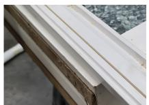
Gently tap the cill into the cill groove, ensuring it sits level and even along the width of the window. We recommend using a piece of softwood or other solid item to protect the paint finish from damage.
