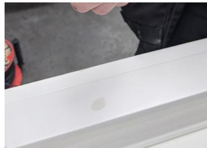
**3** Apply several coats of matched colour Teknos Aquatop 2600 paint over the sanded area of filler. Touch up paint can be partially diluted with a small amount of clean water to achieve a smoother finish. More coats of a diluted paint will be required to cover the damaged area, however this will ensure a much smoother finish.
