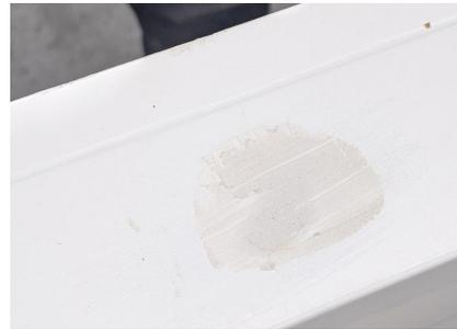
**2** Once fully cured, sand the area of filler smooth with p120 grade sandpaper, taking extra time and care to ensure the filled area is perfectly smooth. This will ensure the best possible repair, leaving a smooth finish ready for the application of paint.
