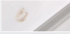
**Prep work:** Firstly, prepare the area, removing any loose, split or flaking sections of the coating by using sandpaper with a p120 grade. Once sanded, clean the area with warm water and a lint free cloth or sponge. Allow the cleaned areas to dry thoroughly before undertaking any coating application.
